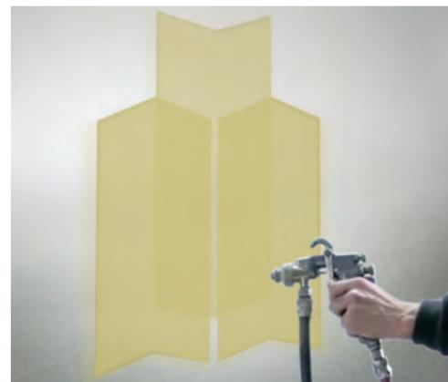
with **vertical** passes with a 50% overlap on each stroke. Leave the fluid pressure the same but lower the air pressure to match the control sample.
